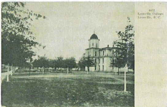
Haynes Auditorium: Prior to the removal of the third floor and cupola
