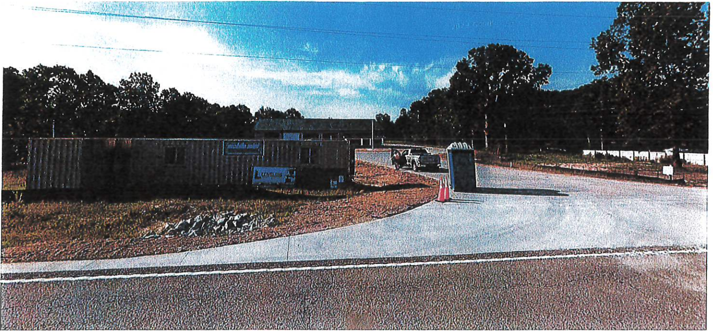
Adjacent Fire Department Facility
