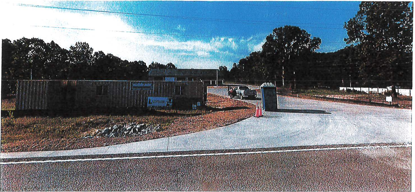
Adjacent Fire Department Facility
